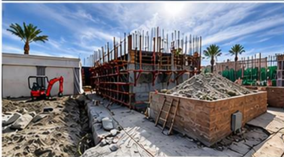
SITE PREPARATION & STRUCTURAL WORK
