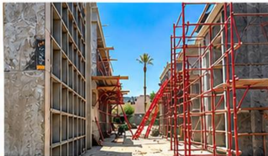
STRUCTURAL STEEL & FRAMING
