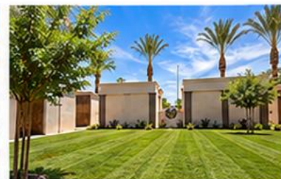
LANDSCAPING & SITE COMPLETION
