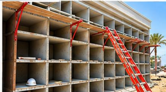
CRYPT WALL CONSTRUCTION
